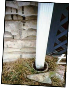
Example of inflow: A downspout connected directly to the sanitary sewer system.
