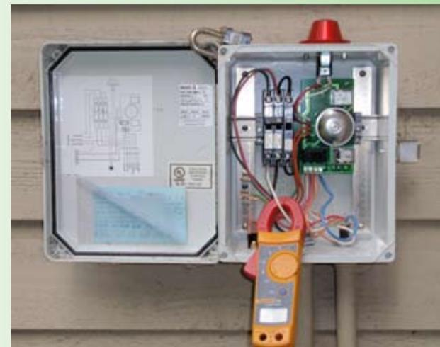
*A District team member will test your grinder pump controller annually to ensure that the alarm functions properly.*
